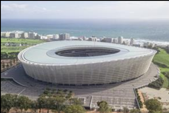
DHL Stadium - Cape Town
