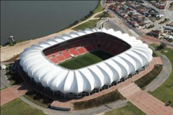
Nelson Mandela Bay Stadium - Port Elizabeth
