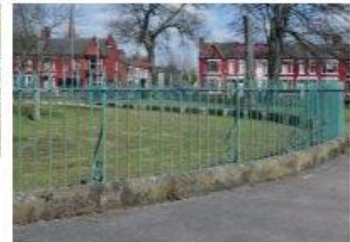
railings, colour, shapes
